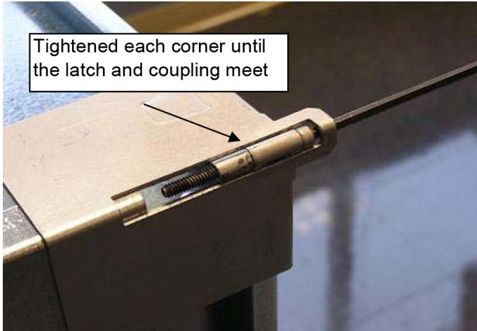
Figure 45: Properly Installed Filter Inside of the Frame
